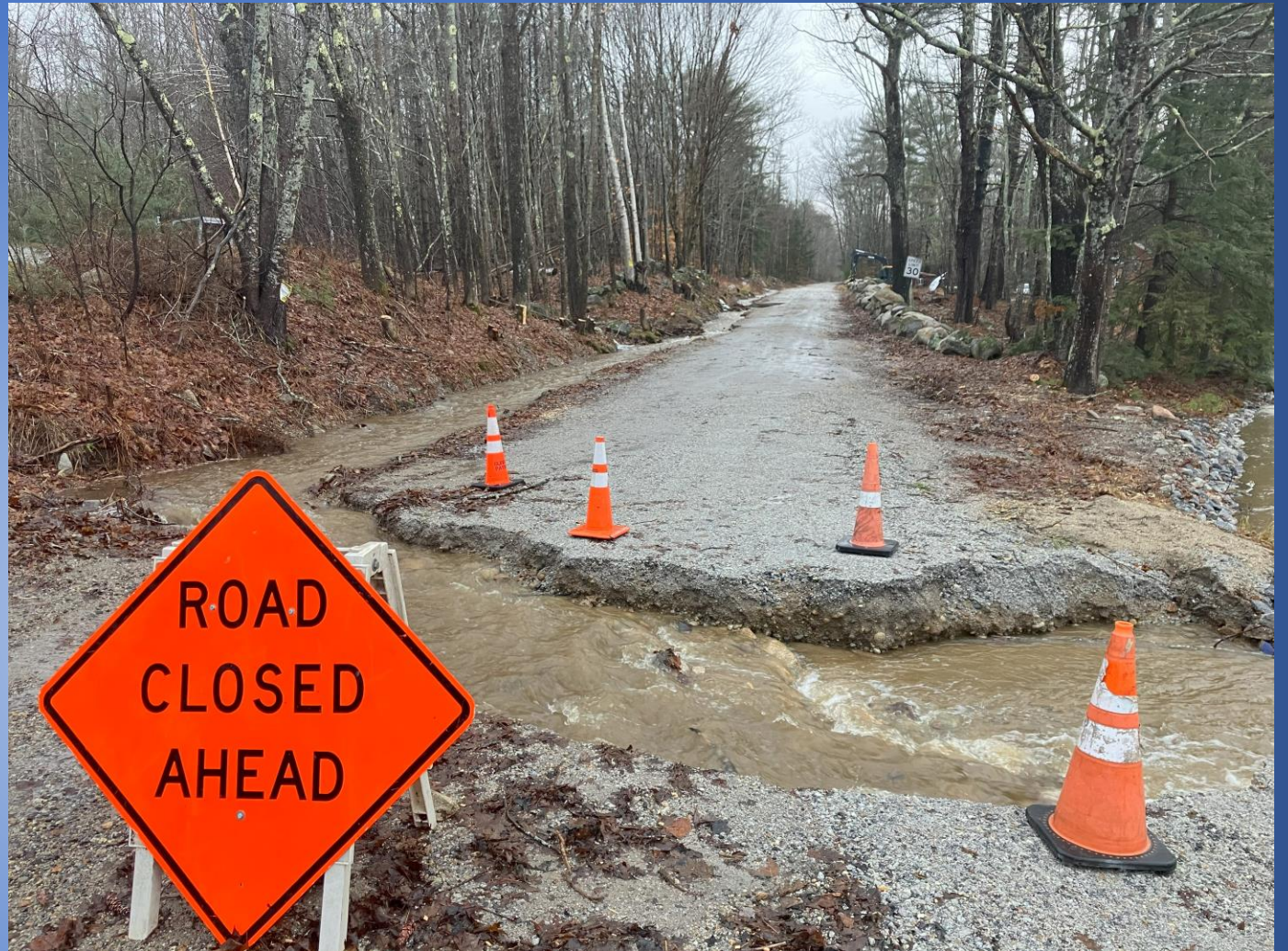
Clogged culverts and ditches
